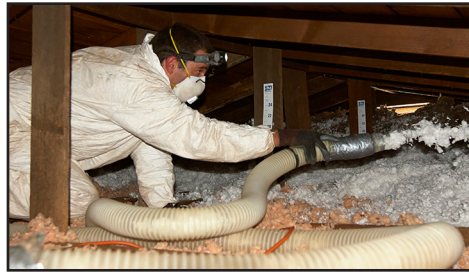
The first step to improving an older home is air sealing and adding insulation to attic spaces. Photo Credit: Bonneville Power Administration
